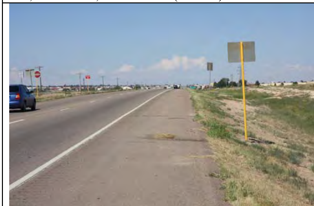
Figure 5. MP 311.0. View west northwest along westbound lanes of US 50 in area mapped as Slocum Alluvium. Lower limestone unit of Smoky Hill Shale Member was mapped just to the west of this area by Scott (1969), but was not observed in the field and may be located outside of the corridor. Photo view UTM 13S, 527921 mE, 4241192 mN (NAD83).
