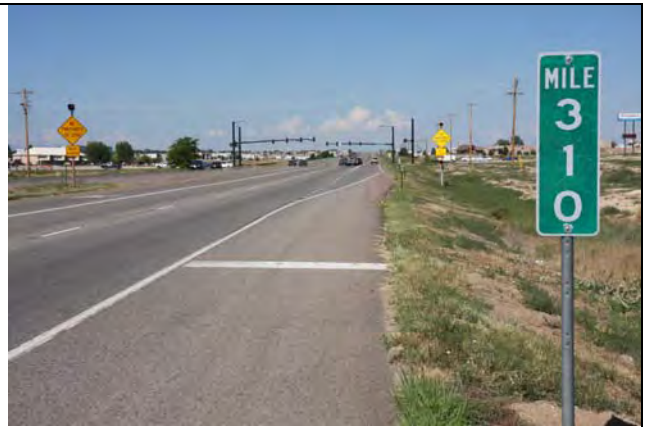
Figure 4. MP 310. View west northwest along US 50 towards western terminus of survey corridor in area mapped as Piney Creek Alluvium. Photo view UTM 13S, 526429 mE, 4241702 mN. (NAD 83).
